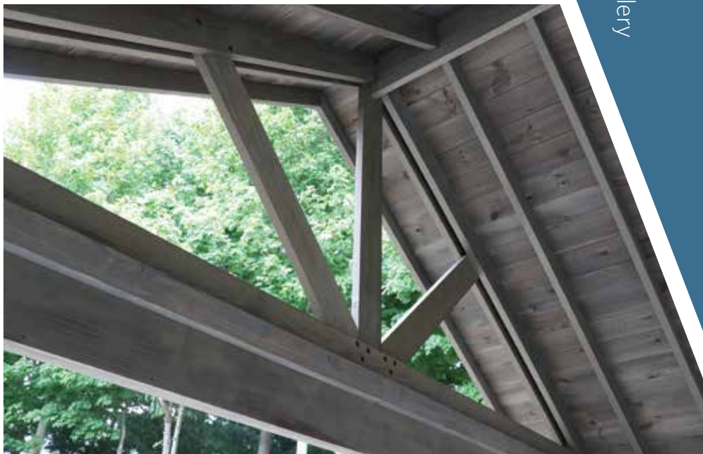
▶ Exposed sheathing pictured.
