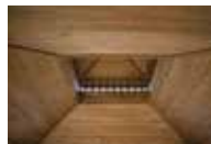
Wood Ceiling Choice of stain color, no paint.
